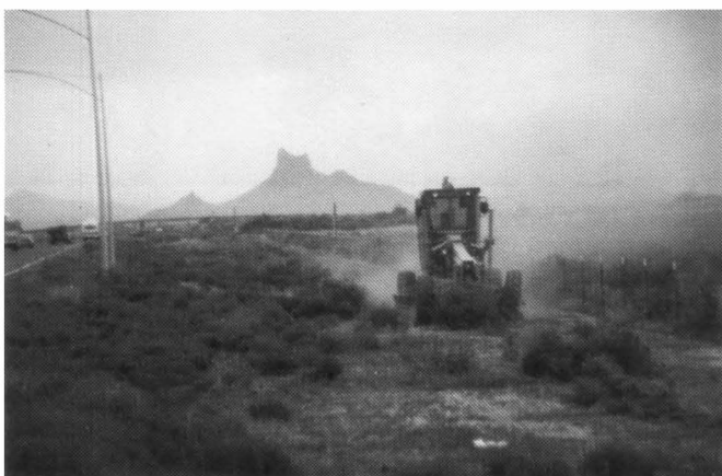
Grading a firebreak along a freeway to prevent forage fires.
