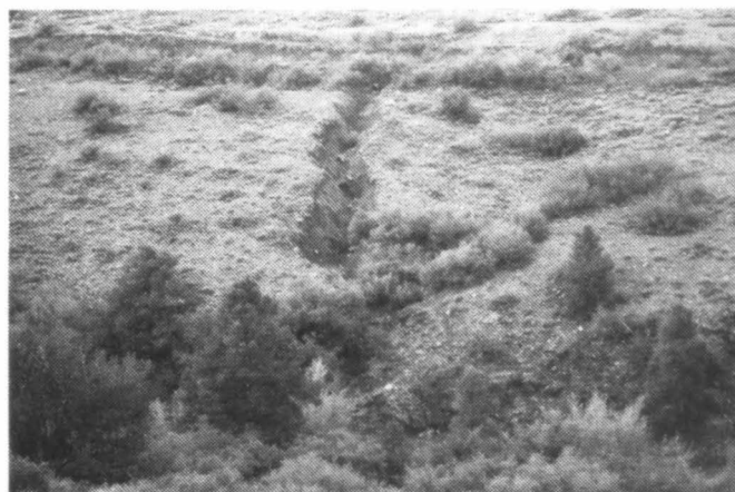
The eroded gash in this hillside is caused by runoff concentrated through a culvert under the ranching road at top.
