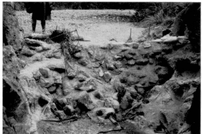
This rock and concrete cattle tank ties into the canyon walls. Note that the basin behind the dam has filled with rocks and gravel.
