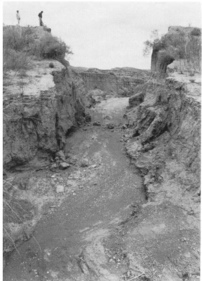
A washed-out stock tank dam on BLM land in central New Mexico. Note the size of the humans at top left.
