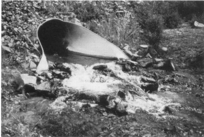
Culverts impede the movement of aquatic life, pervert drainage patterns, cause increased downslope erosion -- and allow destructive roads to exist where they otherwise could not. (Steve Johnson)
