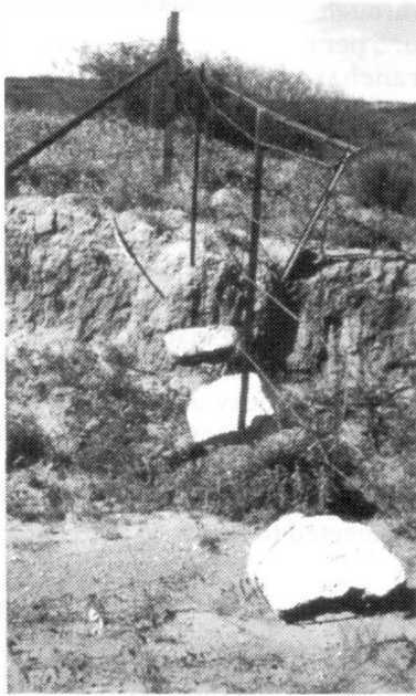
Where fences span drainages and low spots, boulders, logs, or other heavy objects are displaced and wired to strands for stabilization.
