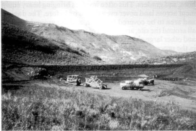
Constructing a large BLM dirt stock tank. (BLM)
